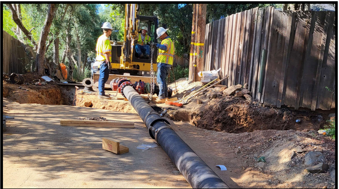
Stratton Way Main Replacement, Auburn
