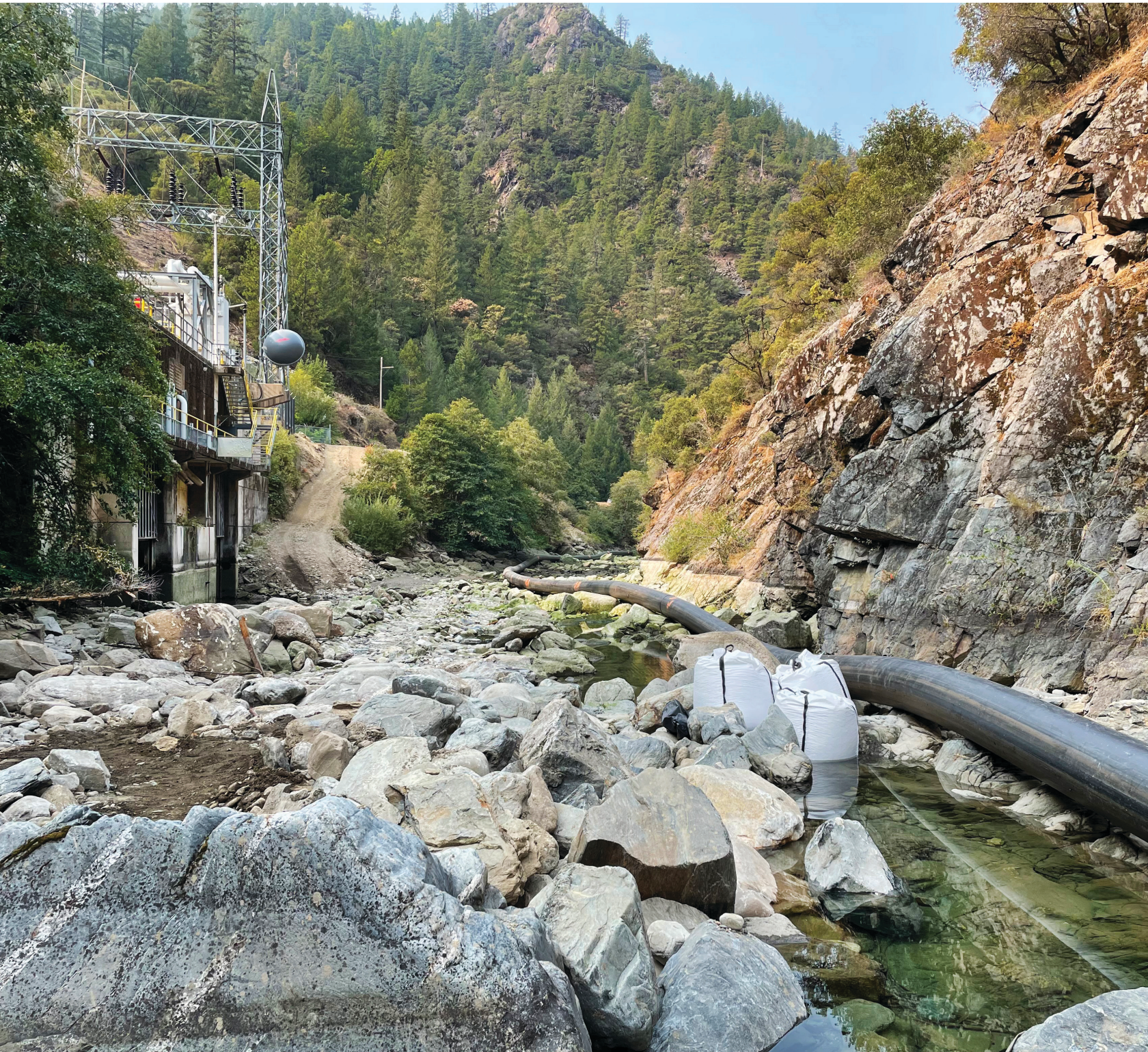
Middle Fork Interbay - Powerhouse Tailrace (Dewatered)
