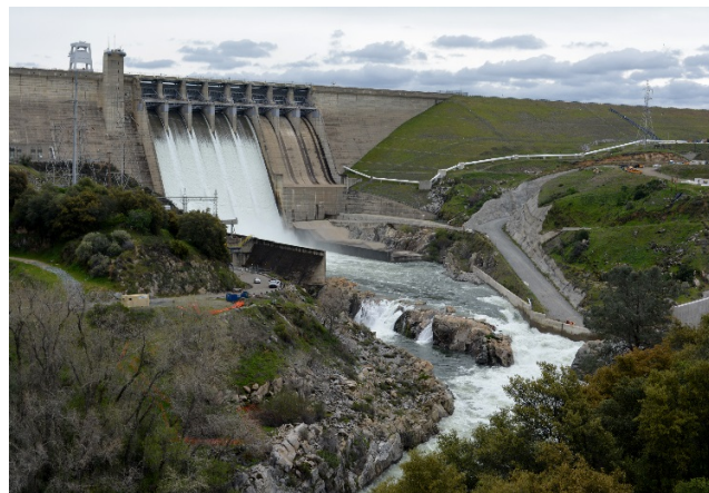
Although drought in California remained, Folsom Reservoir made releases in 2016 to maintain flood space (March 28, 2016).
