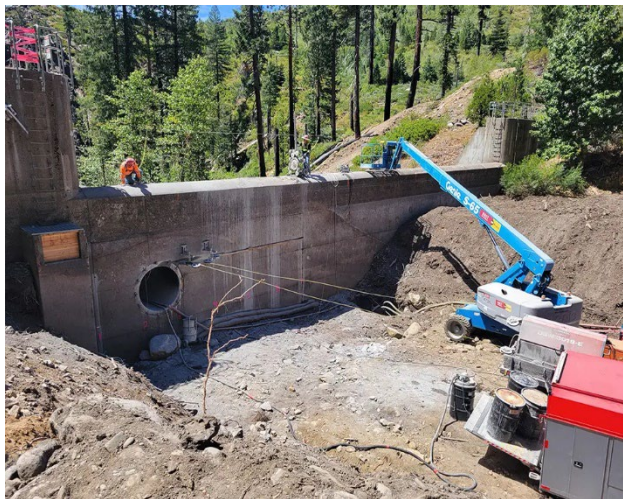
Duncan Creek Diversion Dam
