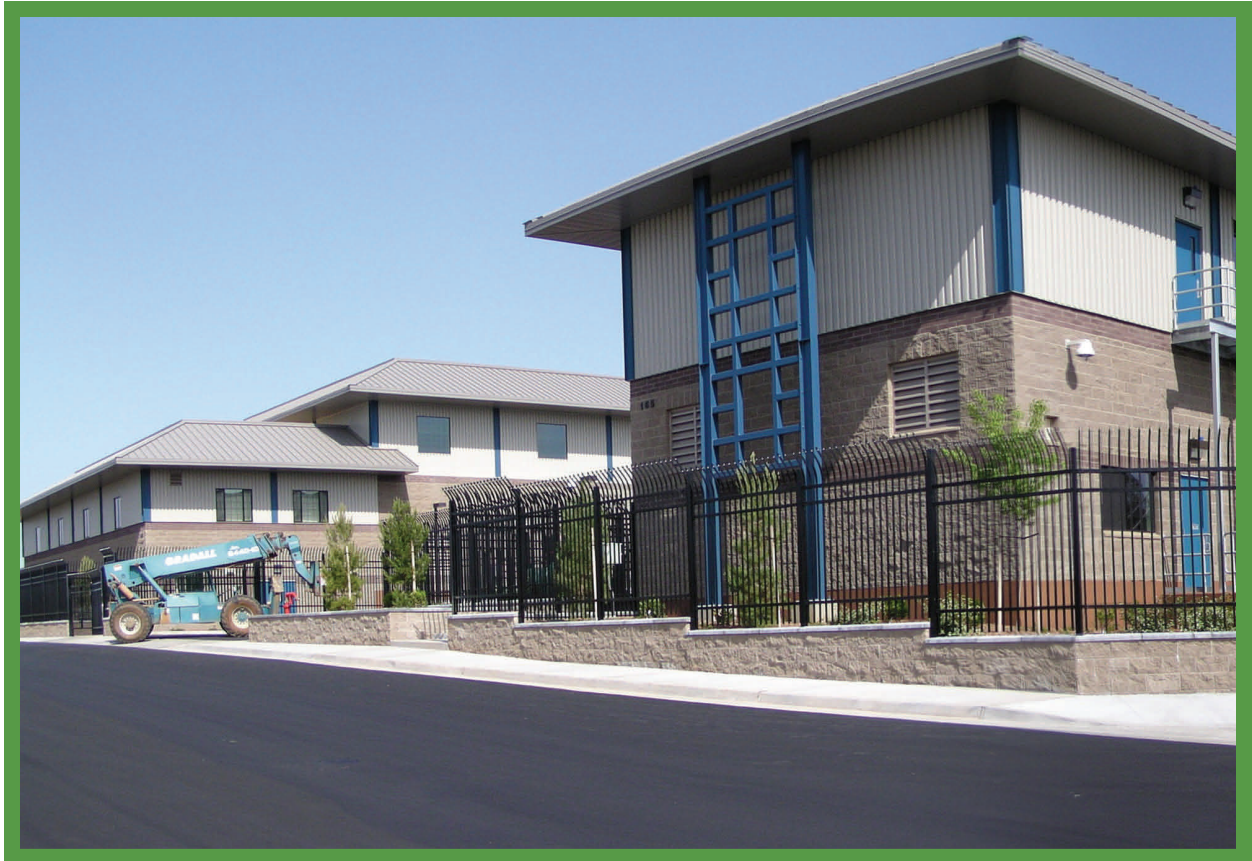
Auburn Water Treatment Plant 8 Million Gallons Per Day (MGD)
