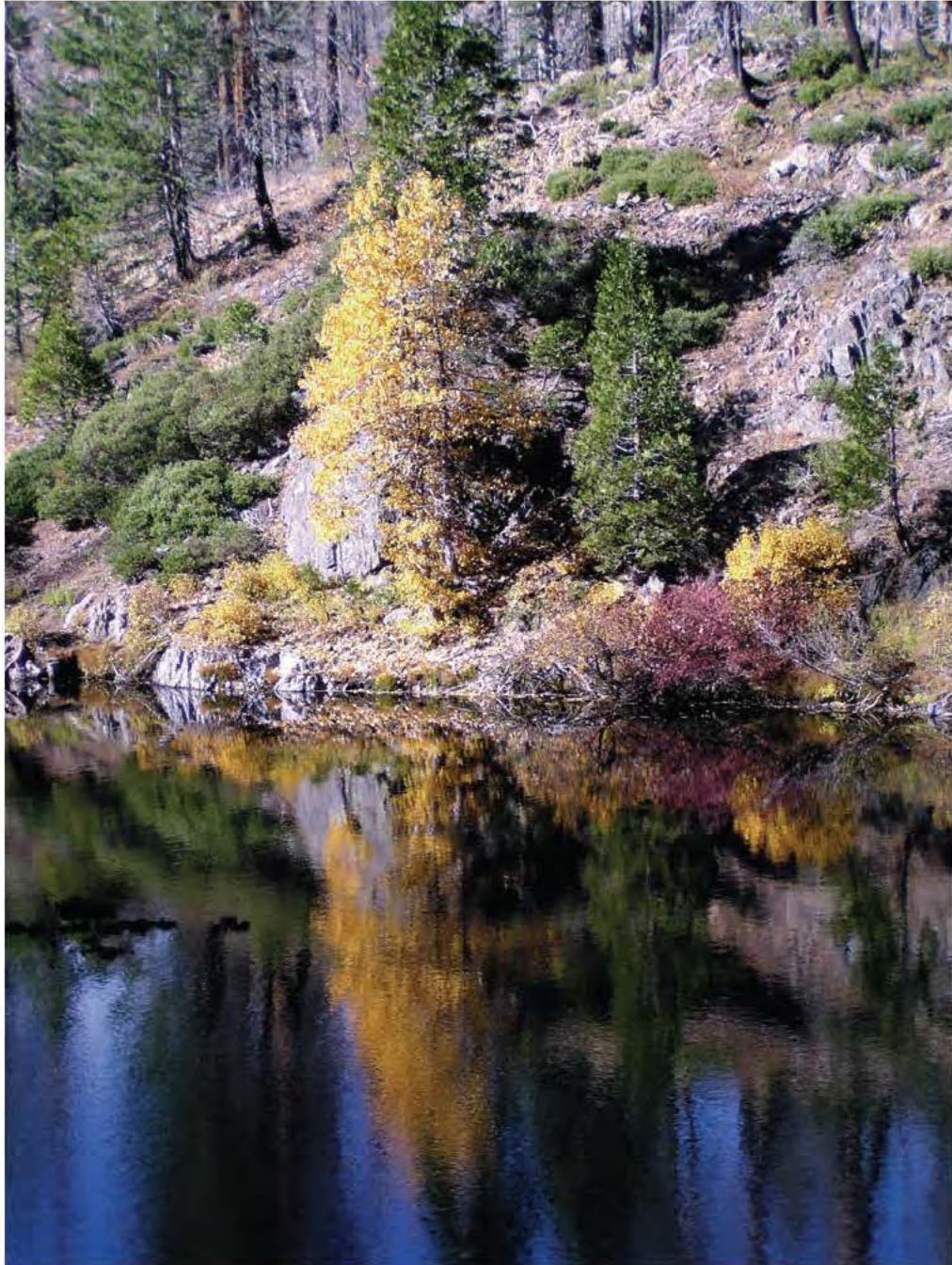
Duncan Diversion Dam
