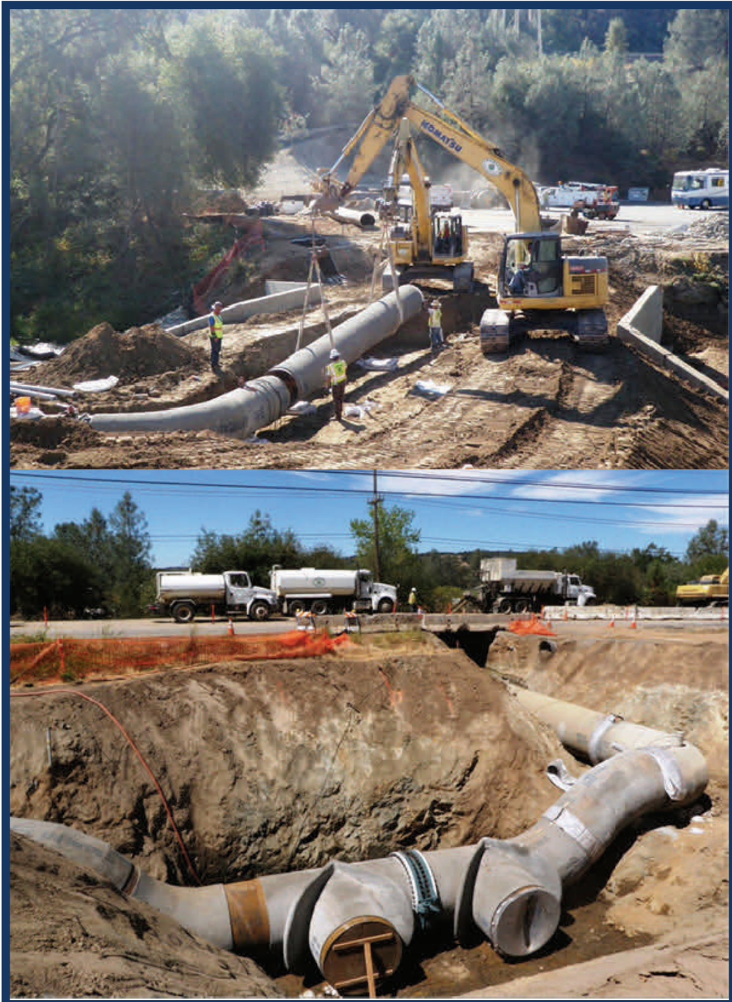
Ophir Road Pipelines Project
