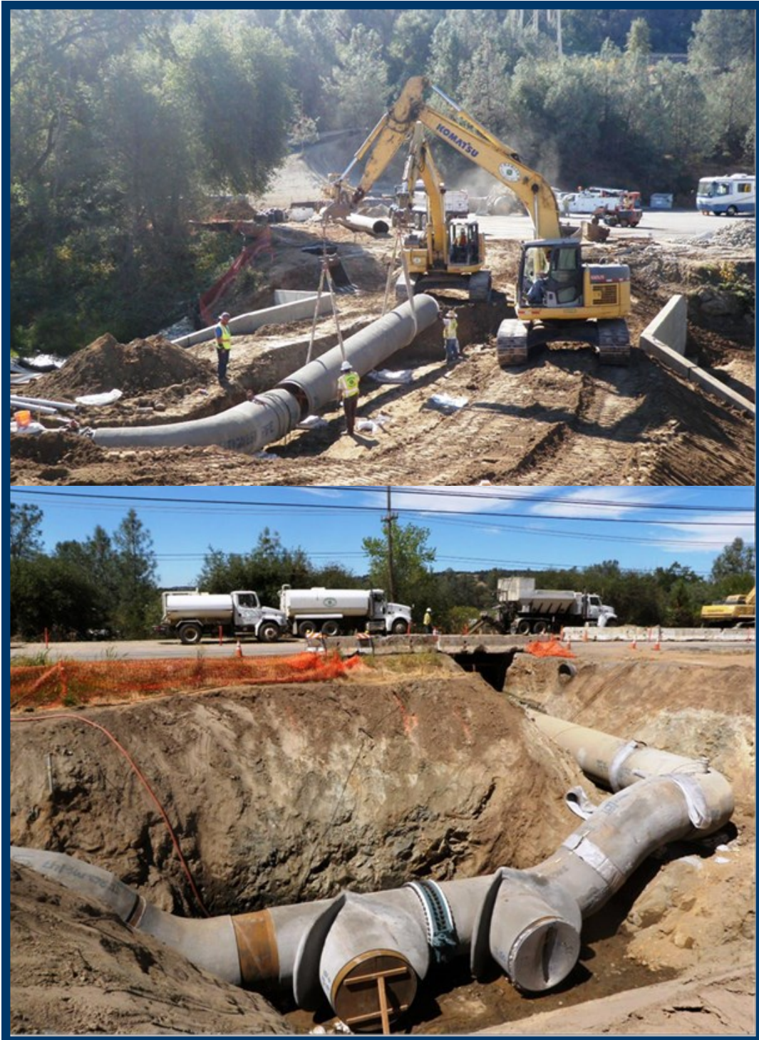
Ophir Road Pipeline Project
