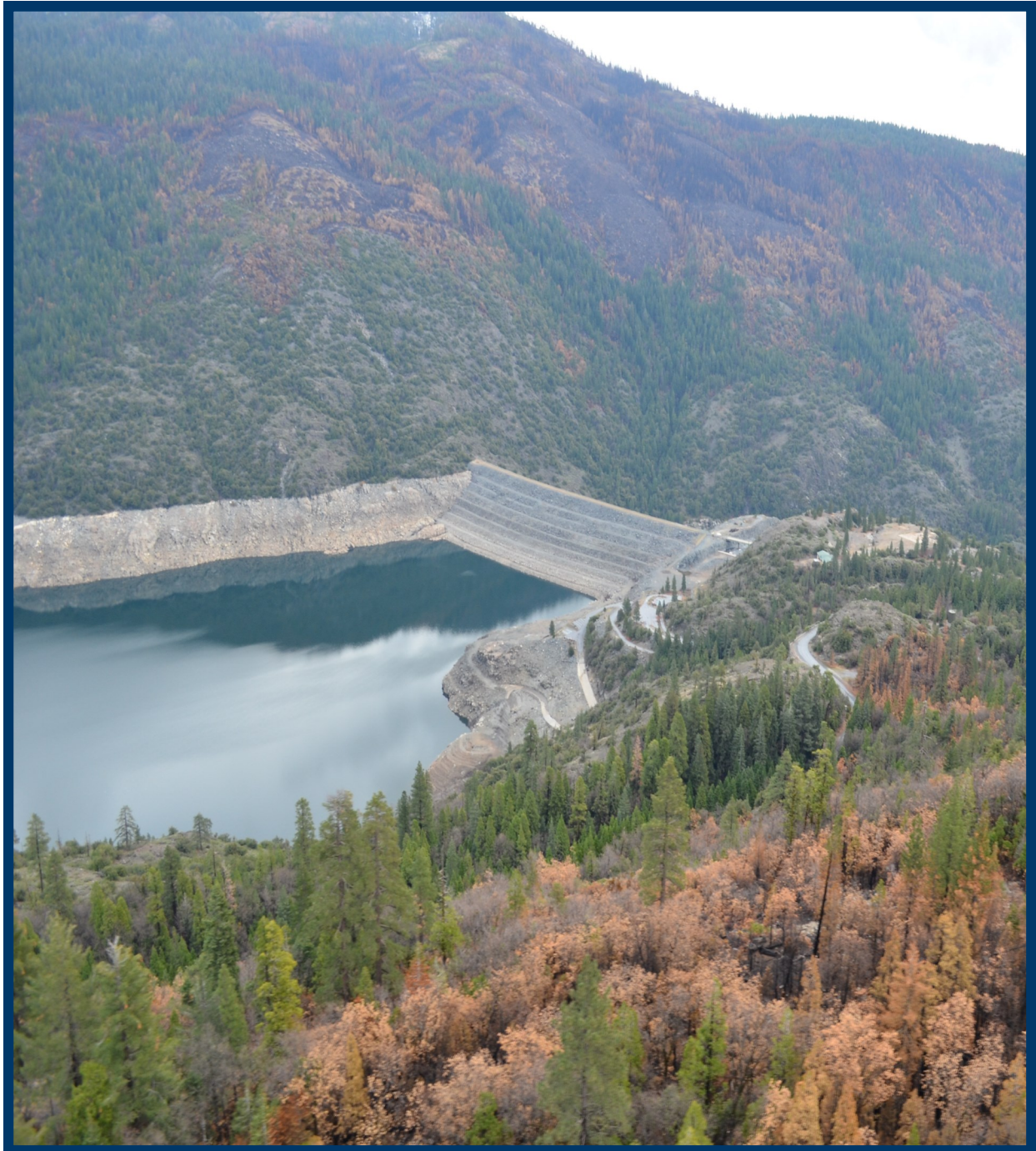
Hell Hole Reservoir with King Fire Damage (foreground and background)
