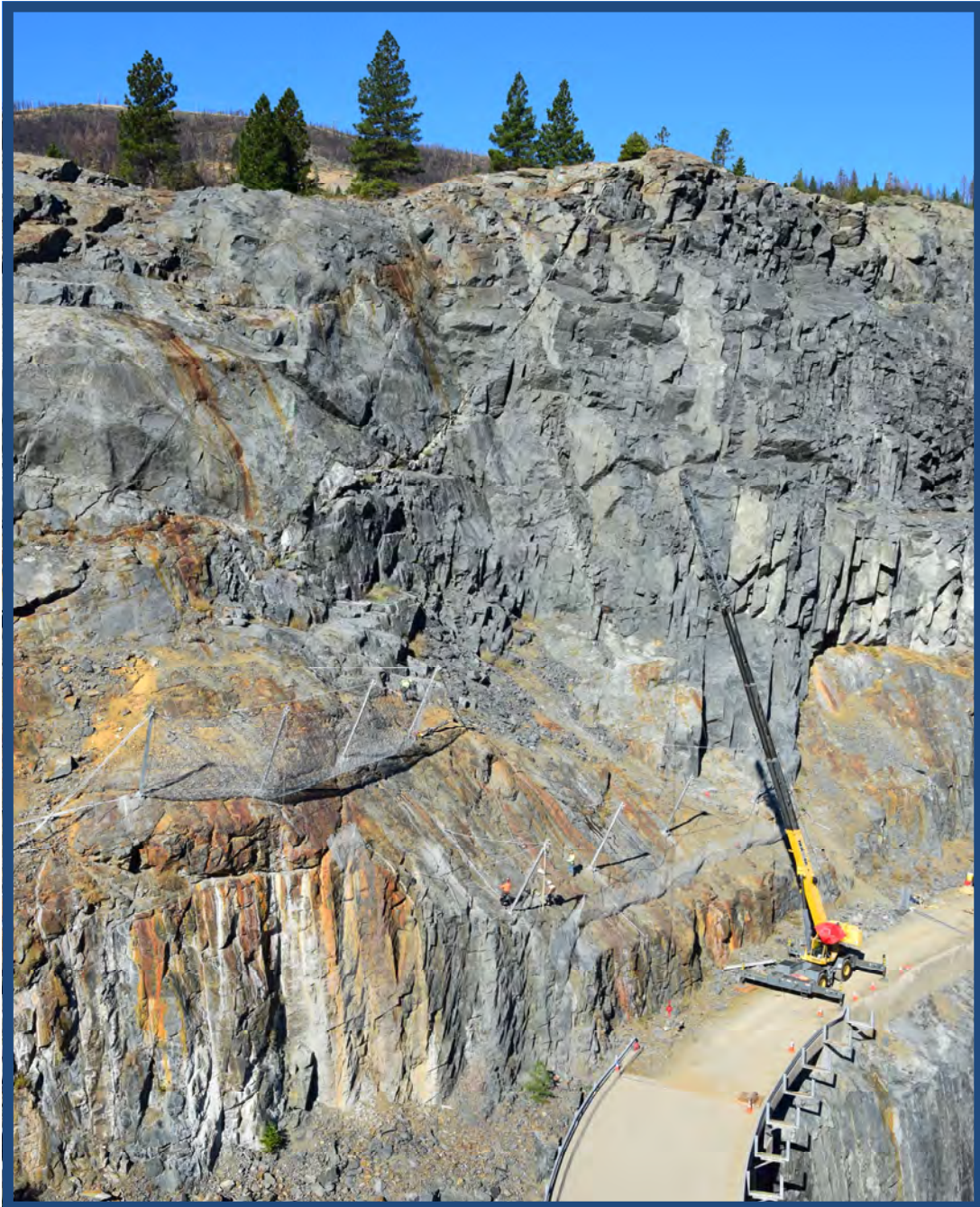
Installation of Hell Hole Dam Spillway Rockfall Barriers
