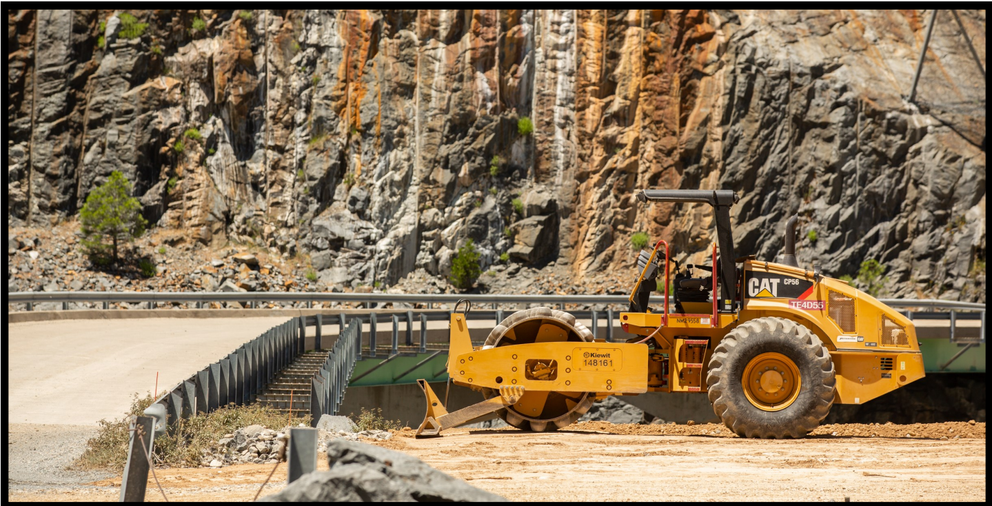
Hell Hole Dam Core Raise Project
