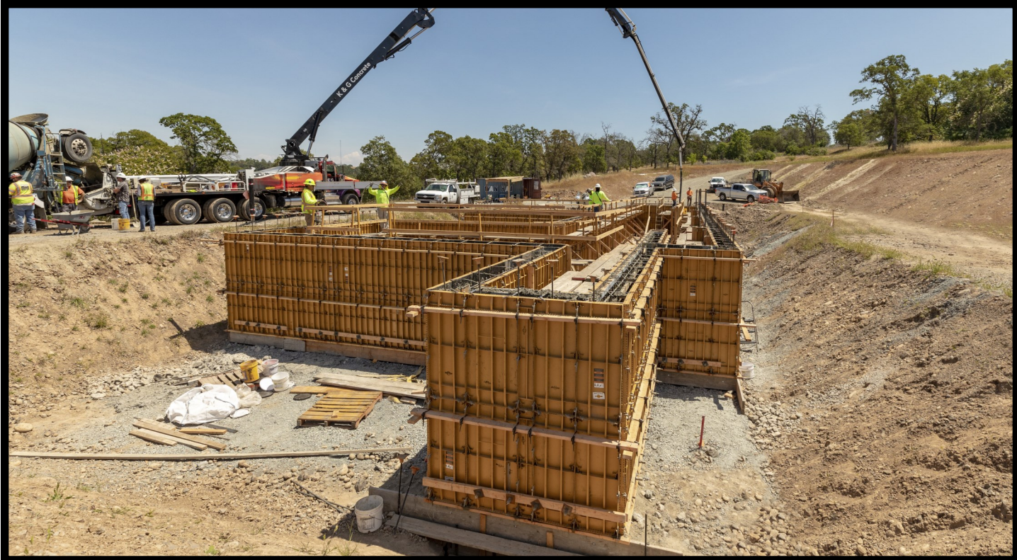
Construction - Lincoln Metering Station
