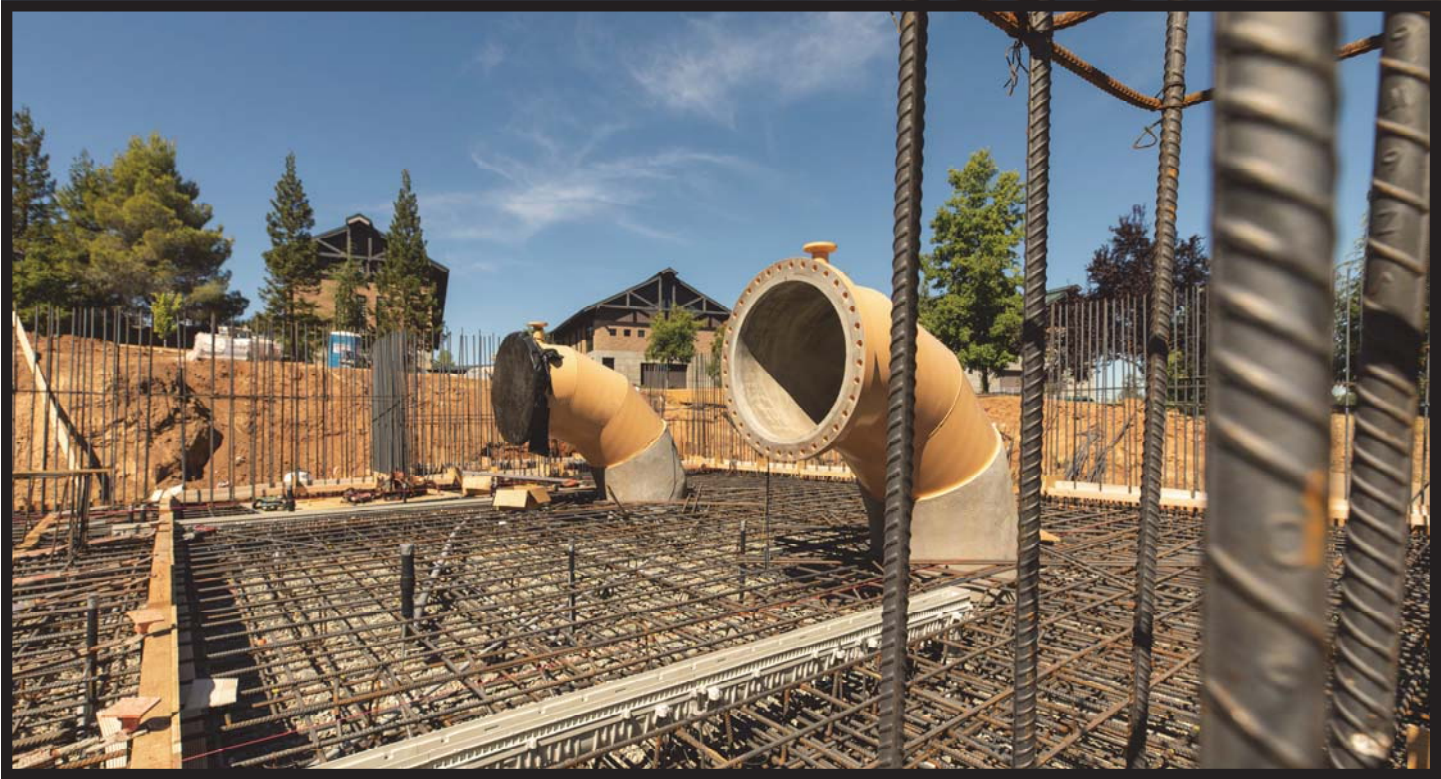
Foothill Raw Water Pipeline Project
